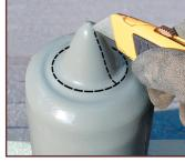
Insert a utility knife in the top cone, cut down to feel the inside edge of the pipe. Use the inside edge as a guide to carefully cut out and remove the cone.
