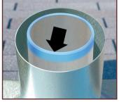
Center base sleeve around vent pipe for equal air circulation. Apply solvent weld to top edge and 1/2" down the outside of the PVC pipe.
