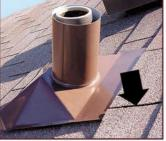
Upper flat section of flange must be completely covered. If necessary, rotate under two rows of shingles and trim to fit.
