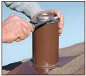
Install the top sleeve. Snap on standard cap or tighten the clamp on the frost inhibiting cap.
