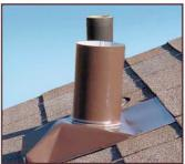
Place new vent pipe flange next to vent pipe and visually check pitch alignment.
