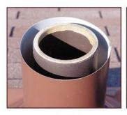
Visually check the base sleeve centered around the vent pipe for equal air circulation.
