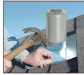
Use embossed guides around perimeter of the base flashing to securely nail the base to the roof.
