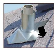
Upper flat section of the flange must be completely covered. If necessary, rotate under two rows of shingles and trim shingles to fit.
