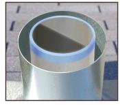
Center base sleeve around vent pipe for equal air circulation. Apply solvent weld to top edge and 1/2" down the outside of the PVC pipe. Slide the Olson Top into position and allow to cure.
