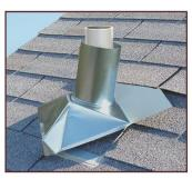
Place the vent flange over the vent pipe and rotate into position under one or more rows of shingles.
