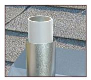
Vent pipe must extend 2" to 5"above base sleeve to allow for roof expansion and contraction. Cut off excess pipe above 5".
