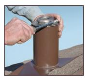
Slide the top sleeve over the base cylinder until the lead seal fits tightly on the vent pipe. Tighten the ring clamp.
