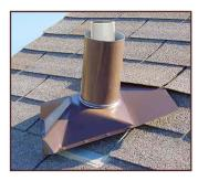
Place the vent flange over the vent pipe and rotate into position under one or more rows of shingles.
