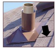
Upper flat section of flange must be completely covered. If necessary, rotate under two rows of shingles and trim shingles to fit.
